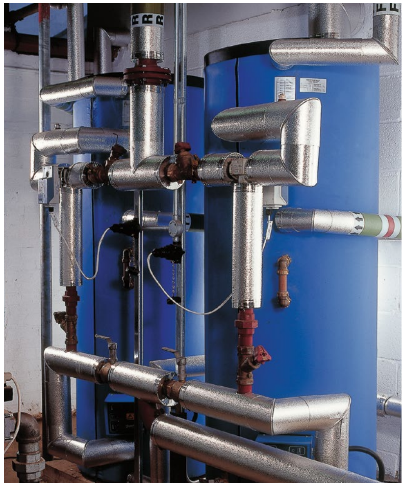
Modular installation of Powerstock calorifiers
